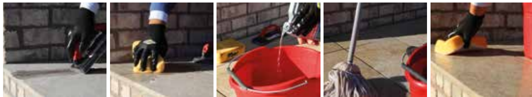
PIC 1. Fill joint with grout.
