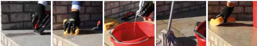
PIC 1. Fill joint with grout.
